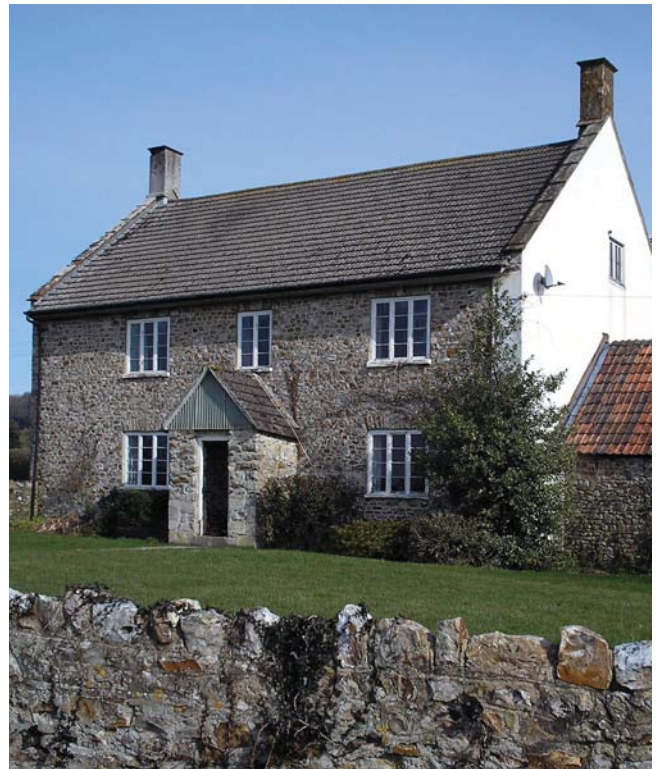
Characteristic 18th century Blackdown Hills symmetrical house, built of chert with gable ends
