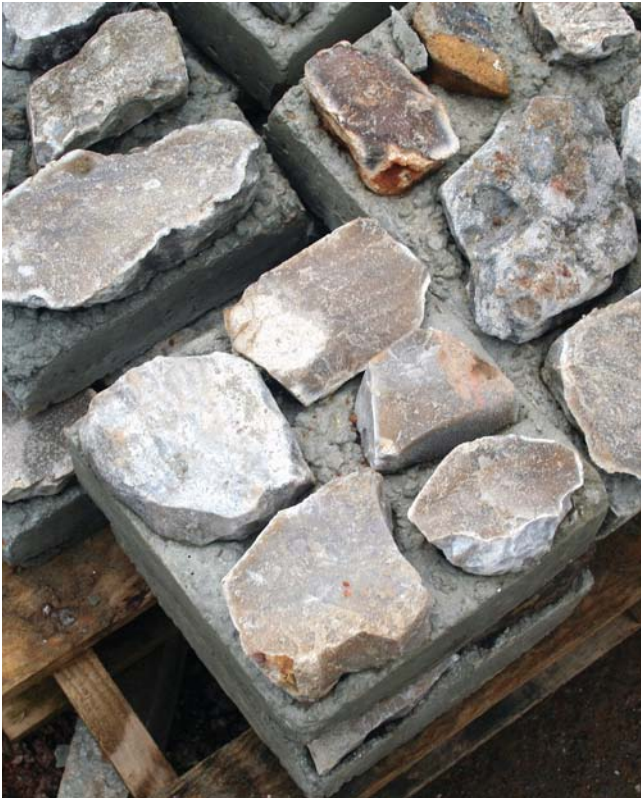
Concrete blocks with in-set flint or chert are available but must be carefully chosen and handled to avoid a heavily-banded appearance
