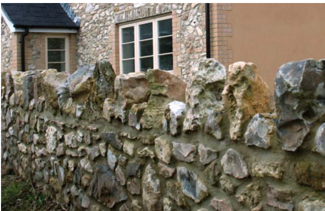
The style of capping used on a wall can contribute much to local distinctiveness
