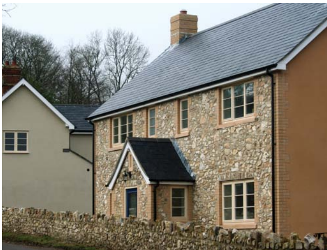
House under construction in the Blackdown Hills
