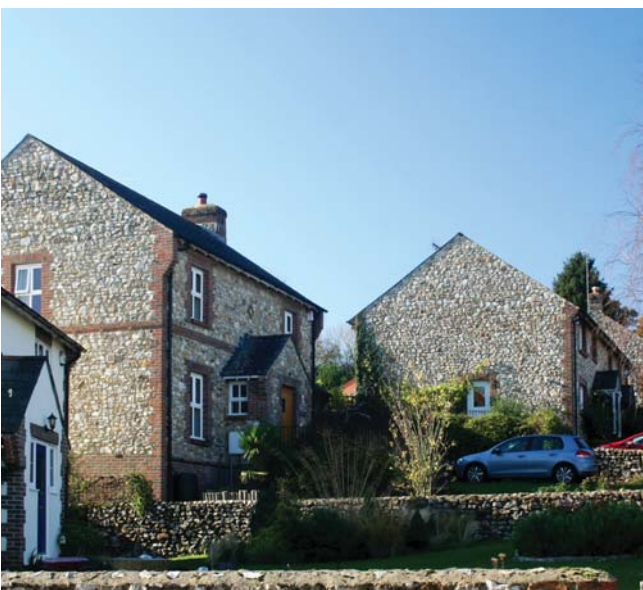
Modern houses, Smallridge, reflecting local building styles and materials
