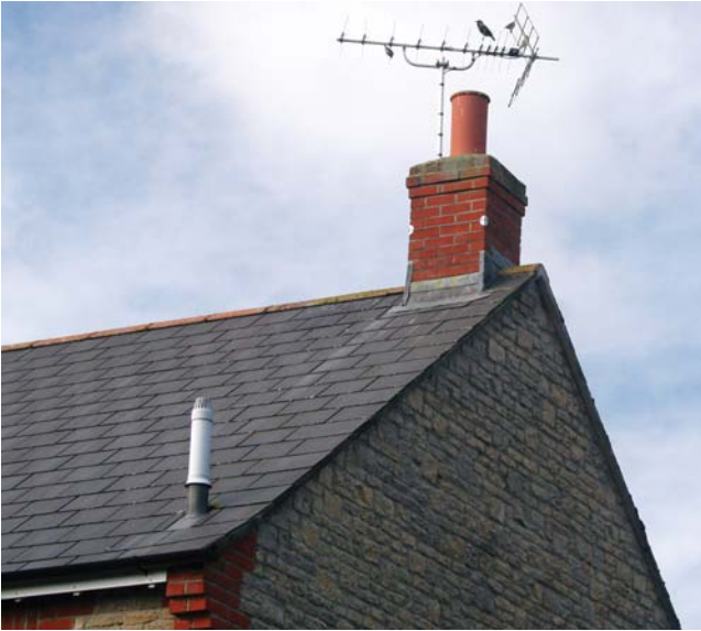
Characteristic gable end roof under modern slate
