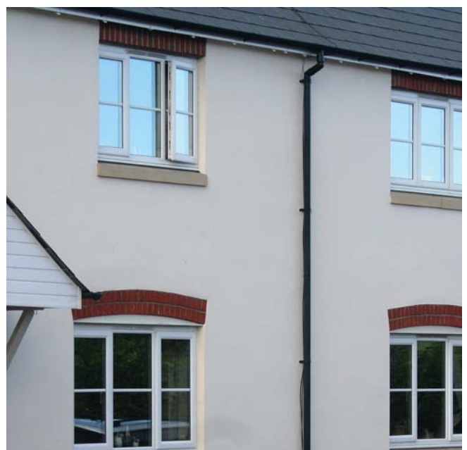
Blackdown Hills' houses tend to have comparatively small windows with multi-paned frames
