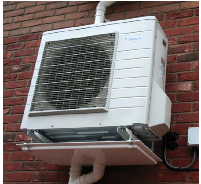
Air source heat pumps are mounted directly on an external wall to make use of the ambient air as a heat source
