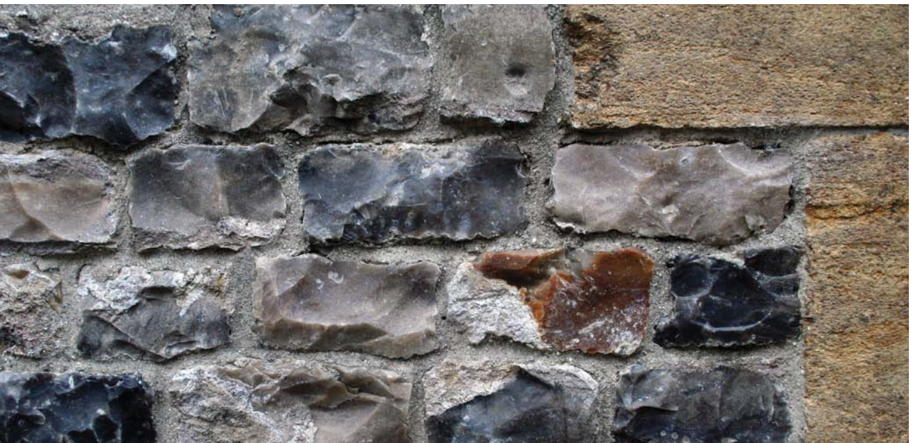
Flint with stone detailing, typical building materials in the Blackdown Hills, in this example laid in courses
